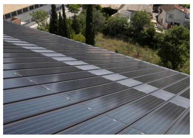
Figure 19 – Example of solar panels on zinc roof where the solar panels are installed between the seams of the zinc
